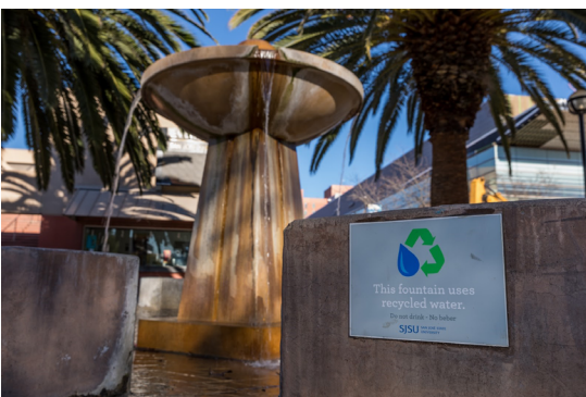
SJSU's first converted fountain includes signage touting its use of recycled water.
