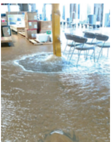
Water bursting from the water main break underneath the foundation.
