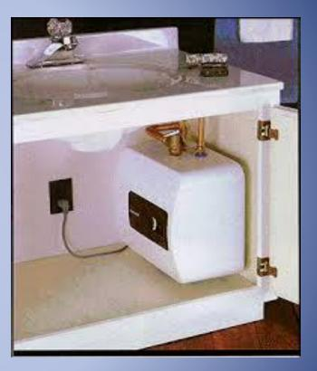
A typical under-the-sink POU water treatment device
