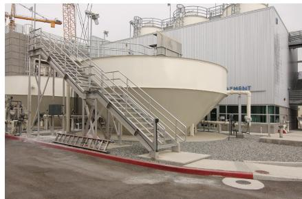
Decarbonator (CO<sub>2</sub> Stripping)
