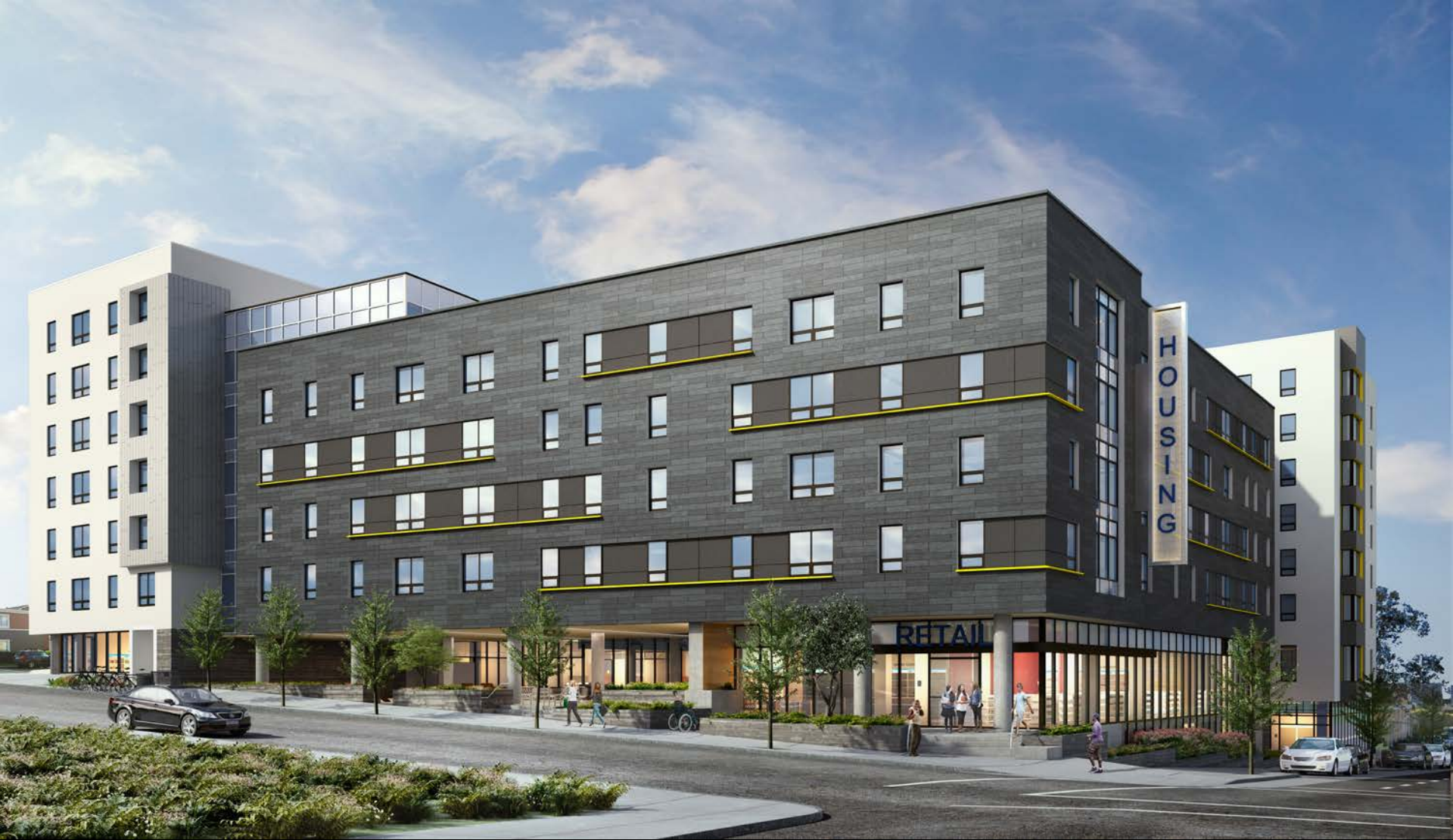
Architect: Gould Evans GC: Build Group, Inc.
