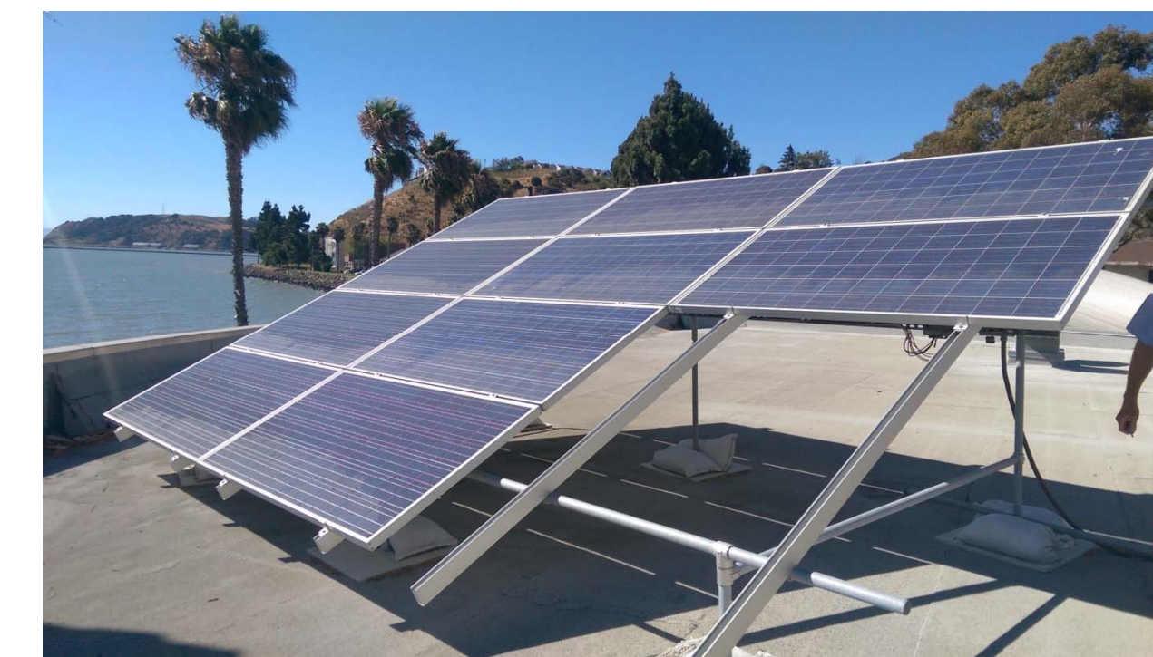
Existing Solar Array on ET Building 10 Panel Solar Array (Trina Solar TSM-280PA14) @ 280W each
