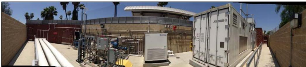
**Storage banks (6k psi)   Compressors   H<sub>2</sub> chiller (-20°C)   Electrolyzer with O<sub>2</sub> vent**
