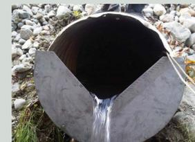
Figure 8. Weir would be temporarily installed on upstream side of Sausal Creek Culverts
