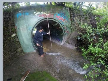
Figure 3. El Centro circular culvert
