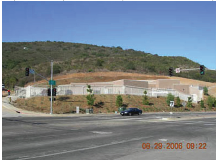
Figure 22. San Diego's Rancho Penasquitos Pressure-Control Facility
