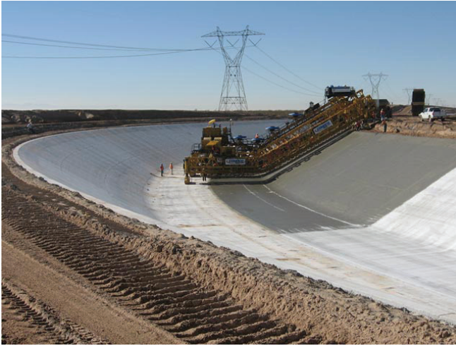
Figure 23. All-American Canal Lining Project.
