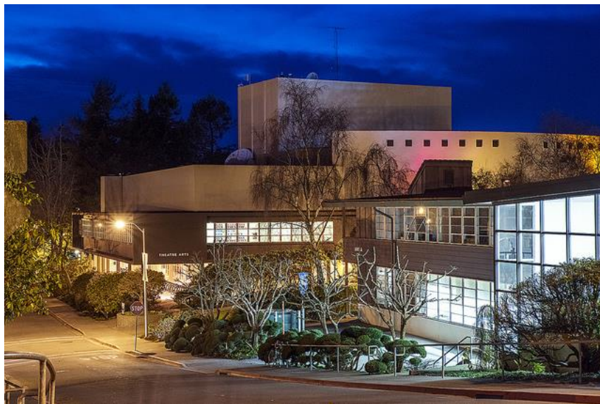
Figure 6 Cal Poly Humboldt Theater Arts renovation
