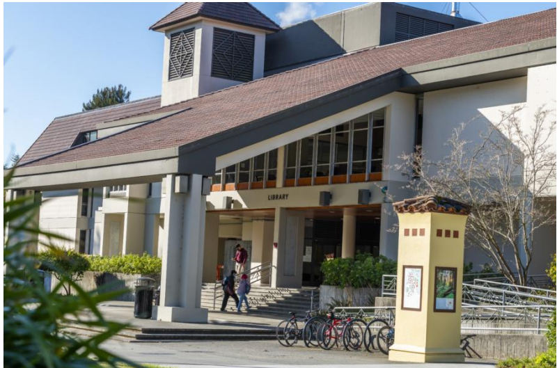
Figure 5 Cal Poly Humboldt Library Renovation
