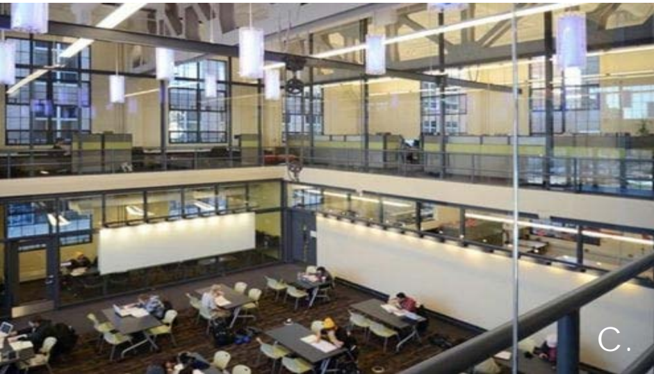
Renovated airplane hangar – University of Minnesota
