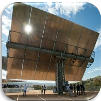
Large solar panels activated at the Cal Poly Pomona Lyle Center on Sept. 30, 2010, making the 16-acre site carbon neutral
