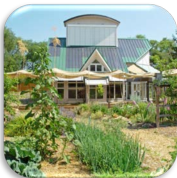
The Environmental Technology Center at Sonoma State is a model for sustainable building techniques and technologies
