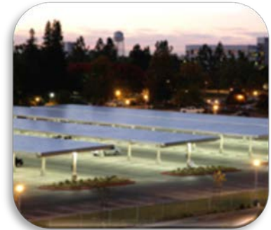
Solar panels covering a CSU Bakersfield parking lot are lit from below at dusk
