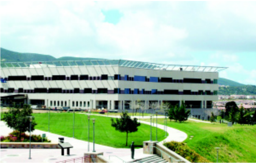
The new Kellogg Library, located at the center of the horseshoe of academic buildings at Cal State San Marcos
