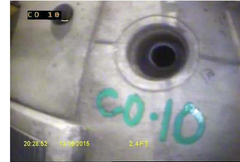
Entry point overview
