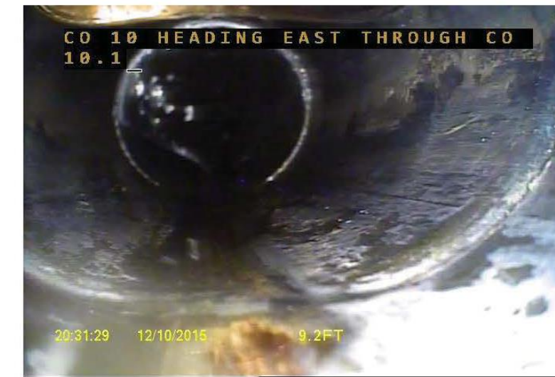
Typical clear line condition
