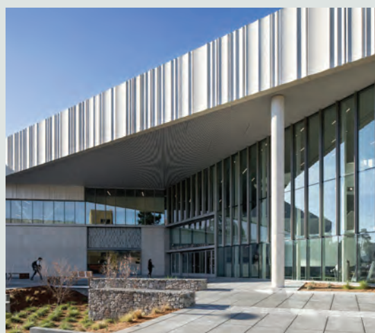
The Mashouf Wellness Center at San Francisco State is on track for LEED Platinum certification.
