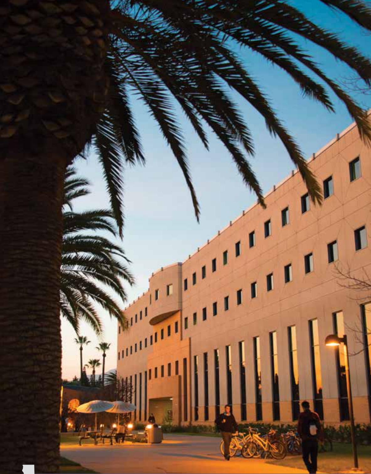
Bookstein Hall at Cal State Northridge
